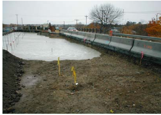
Road Base Over Poor Soil
