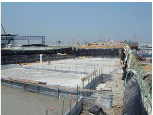
Overpass Approach on soft soil
