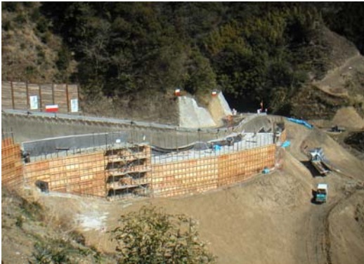
New Road Sub Base
