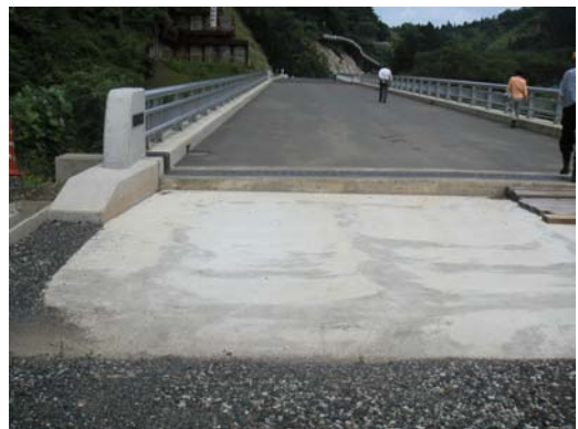
Bridge Abutment to avoid settling
